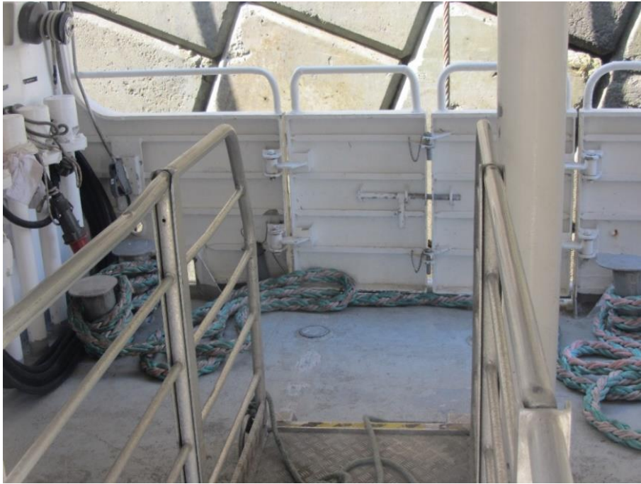
Gates in bulwarks for the gangway to interface with another vessel or the shore
